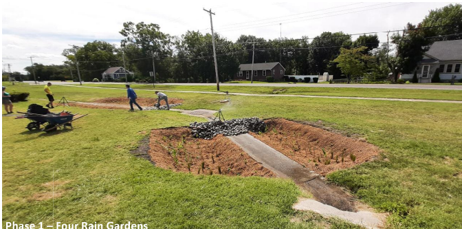
Pittsgrove Middle School, Pittsgrove NJ - In the summer 4 Rain Gardens were installed in an existing detention basin and sections of the low-flow concrete channel were removed to promote water detention.
