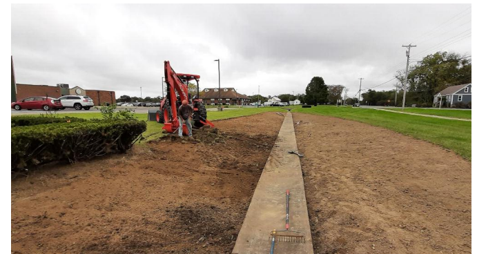
Pittsgrove Middle School, Pittsgrove NJ - In the summer 4 Rain Gardens were installed in an existing detention basin and sections of the low-flow concrete channel were removed to promote water detention.
