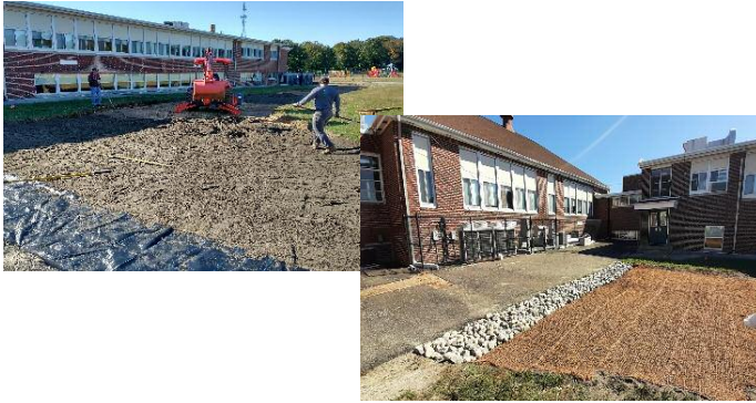
Olivett Elementary School, Elmer NJ - A 4,125 square foot Bioswale spanning 225 feet in length was installed in the courtyard area..
