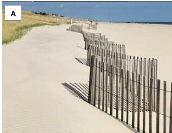
Figure 8A, B. Examples of dune fences with sand accumulation.
