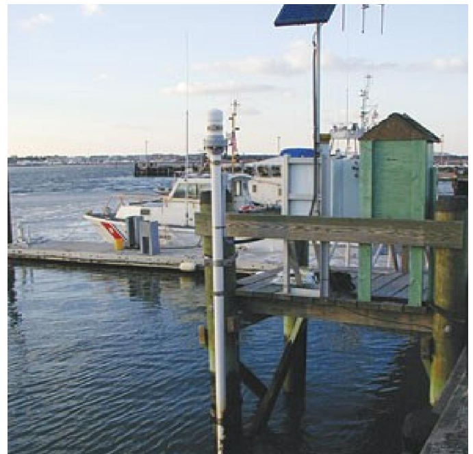
Tidal gauge - the white pipe contains tide level detection equipment.
