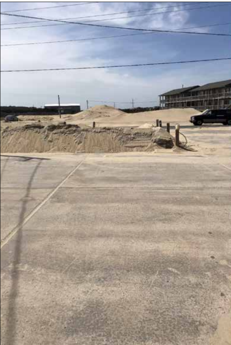
Figure 8. Temporary sand pile along the road to keep sand out of the streets (left). Temporary sand piles on the beach front to protect the houses from overwash (right).
