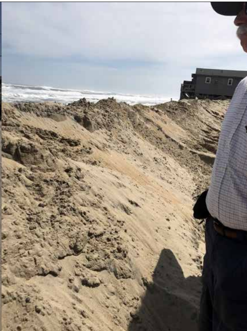
Figure 8. Temporary sand pile along the road to keep sand out of the streets (left). Temporary sand piles on the beach front to protect the houses from overwash (right).
