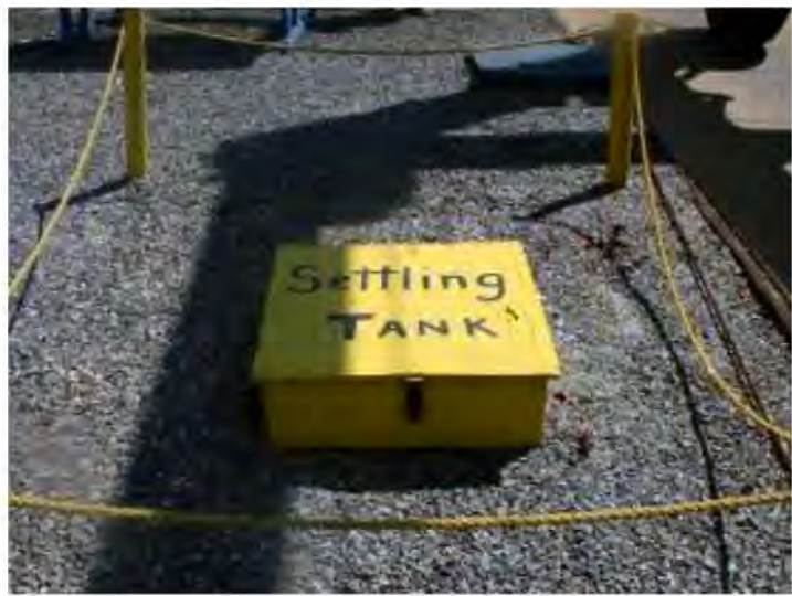
Wash wastewater is collected in an underground storage tank where solids are settled.
