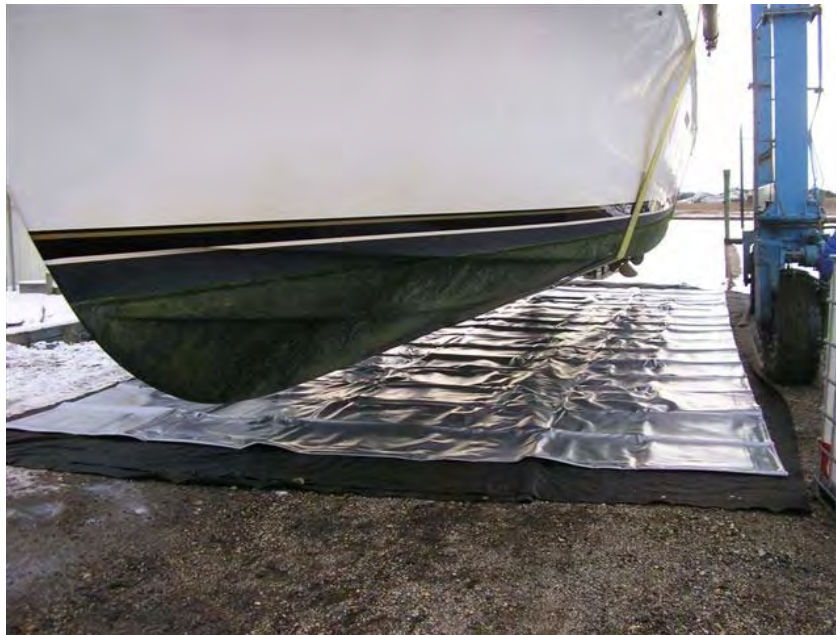
Figure 2: Polyvinyl chloride (PVC) wash pad (19 feet by 45 feet by 50 mil thick)
