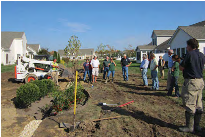
The Delaware workshop exercises included the creation of a functioning rain garden.
