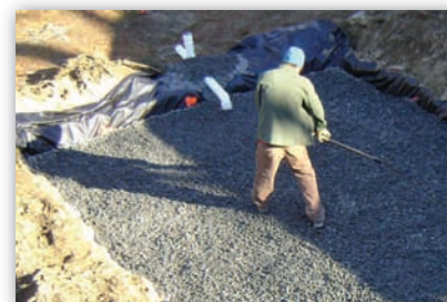
Ben Pearson adds gravel to the engineered rain garden on the GCU campus.
