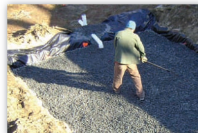
Ben Pearson adds gravel to the engineered rain garden on the GCU campus.
